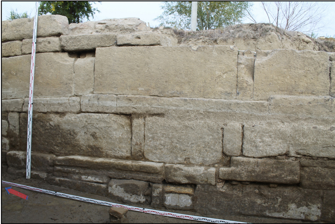
Fig. 7. The Rubas Fortification of the 6th c. Wall 2. Western facade. Central section. View from the west. Photo 2017
