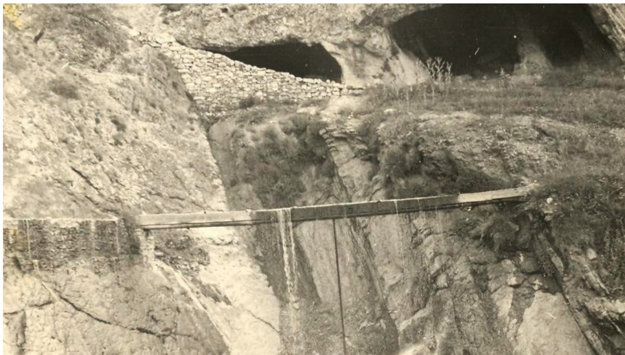
Fig. 15. Transfer of water through the gorge. Canal tunnels at the top. Gergebil village. Photo by M. Aglarov, 1967
