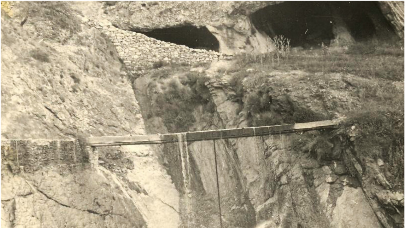
Fig. 15. Transfer of water through the gorge. Canal tunnels at the top. Gergebil village. Photo by M. Aglarov, 1967
