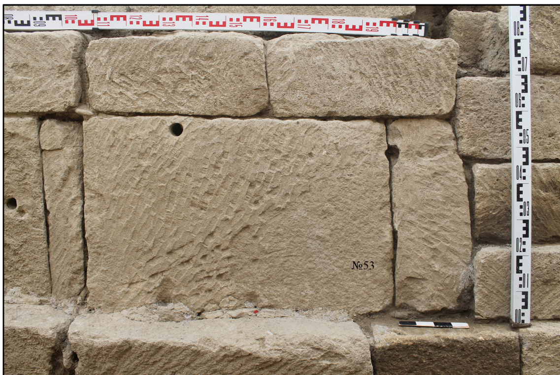
Fig. 8. Monumental architectural structure on river Rubas. Structure No. 2. Eastern façade. Block No. 53. View from east.
