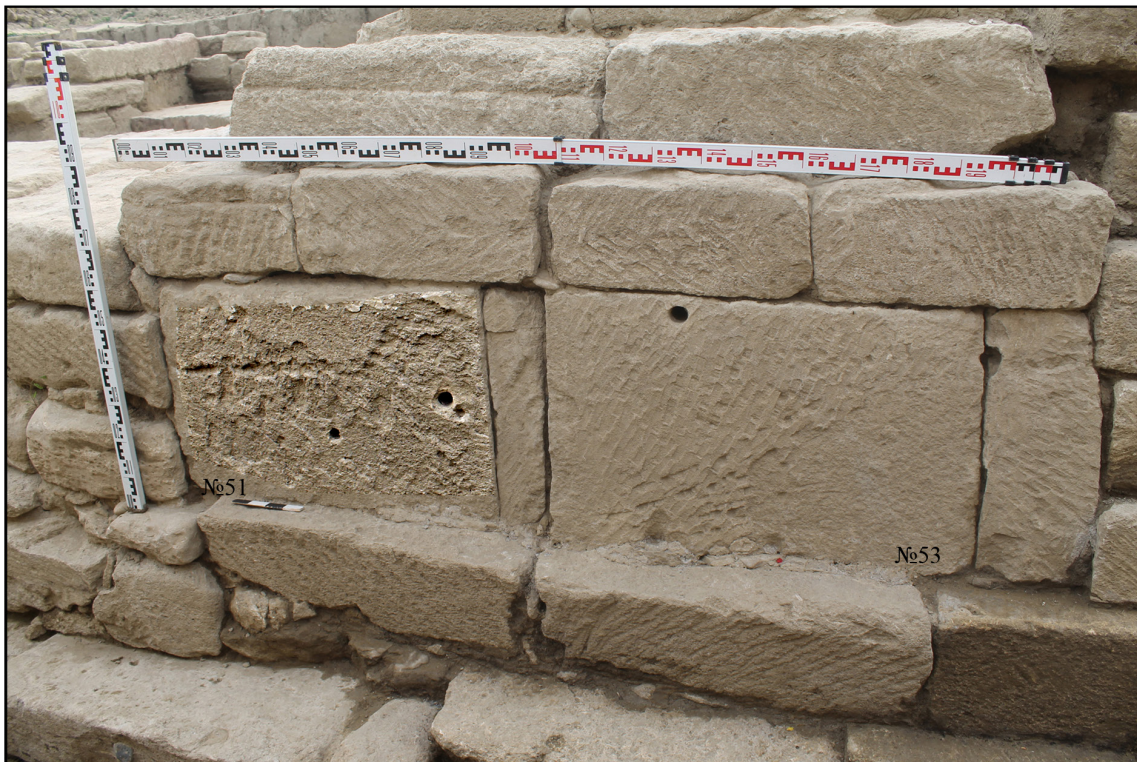
Fig. 7. Monumental architectural structure on river Rubas. Structure No. 2. Eastern façade. Blocks Nos. 51-53. View from east
